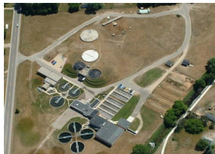
Wastewater Treatment Facility
