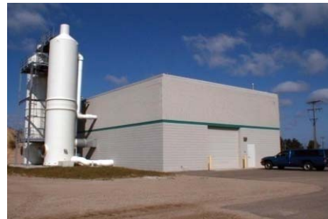
LDFA Water Treatment Facility
