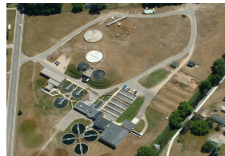
Wastewater Treatment Facility
