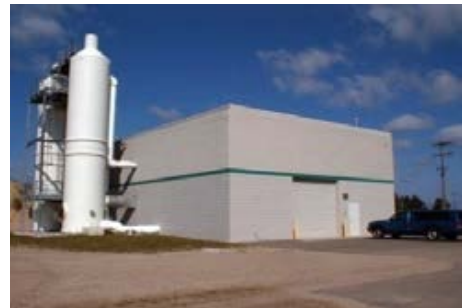
LDFA Water Treatment Facility
